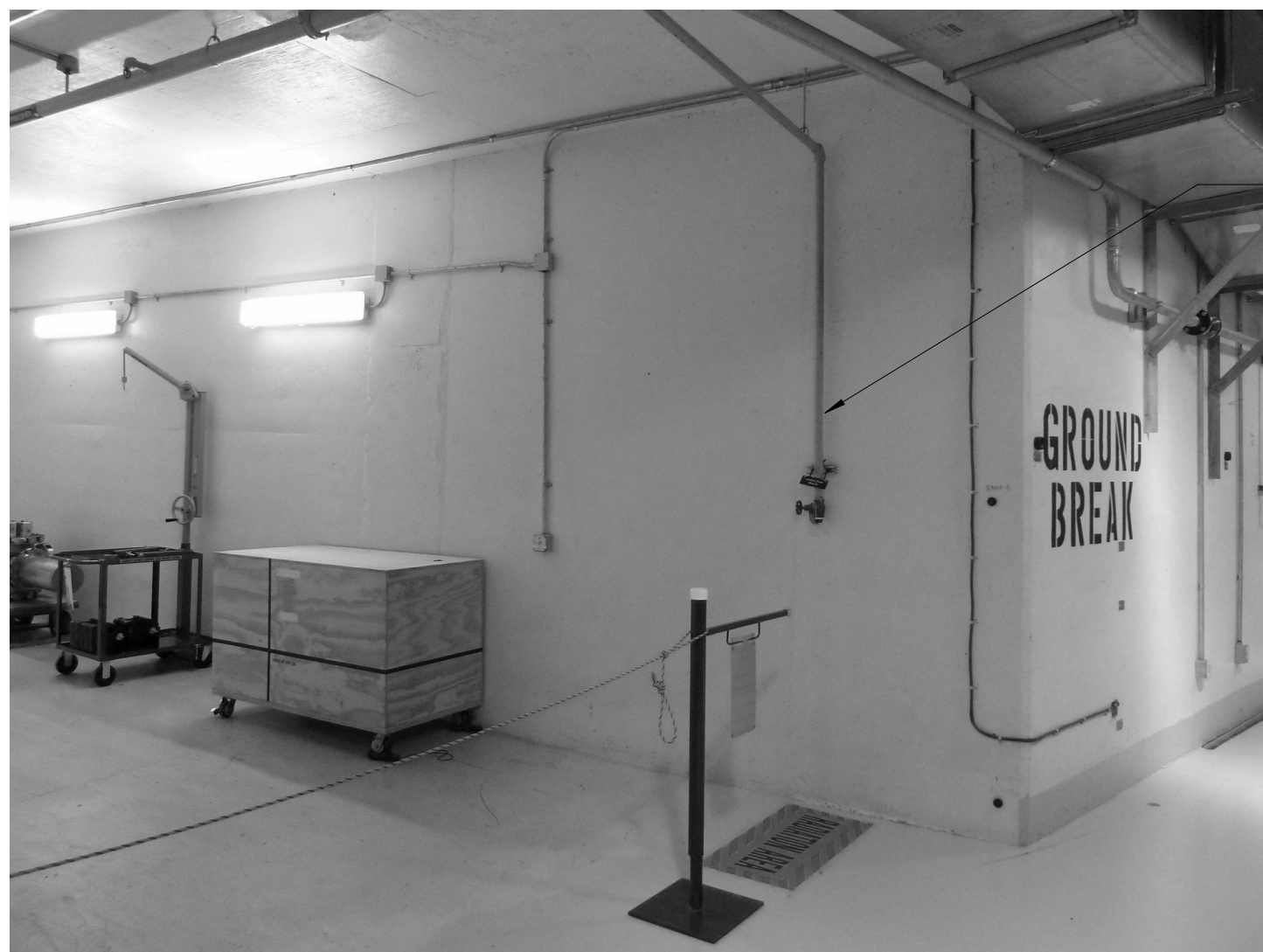
4 FIRE PROTECTION PIPING RELOCATION NTS
