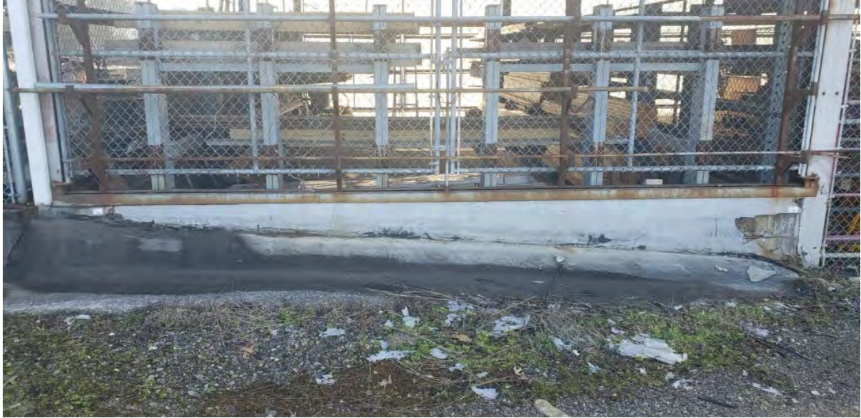
Bldg. 7070, SID13979; roof flashing material at base of bldg.
