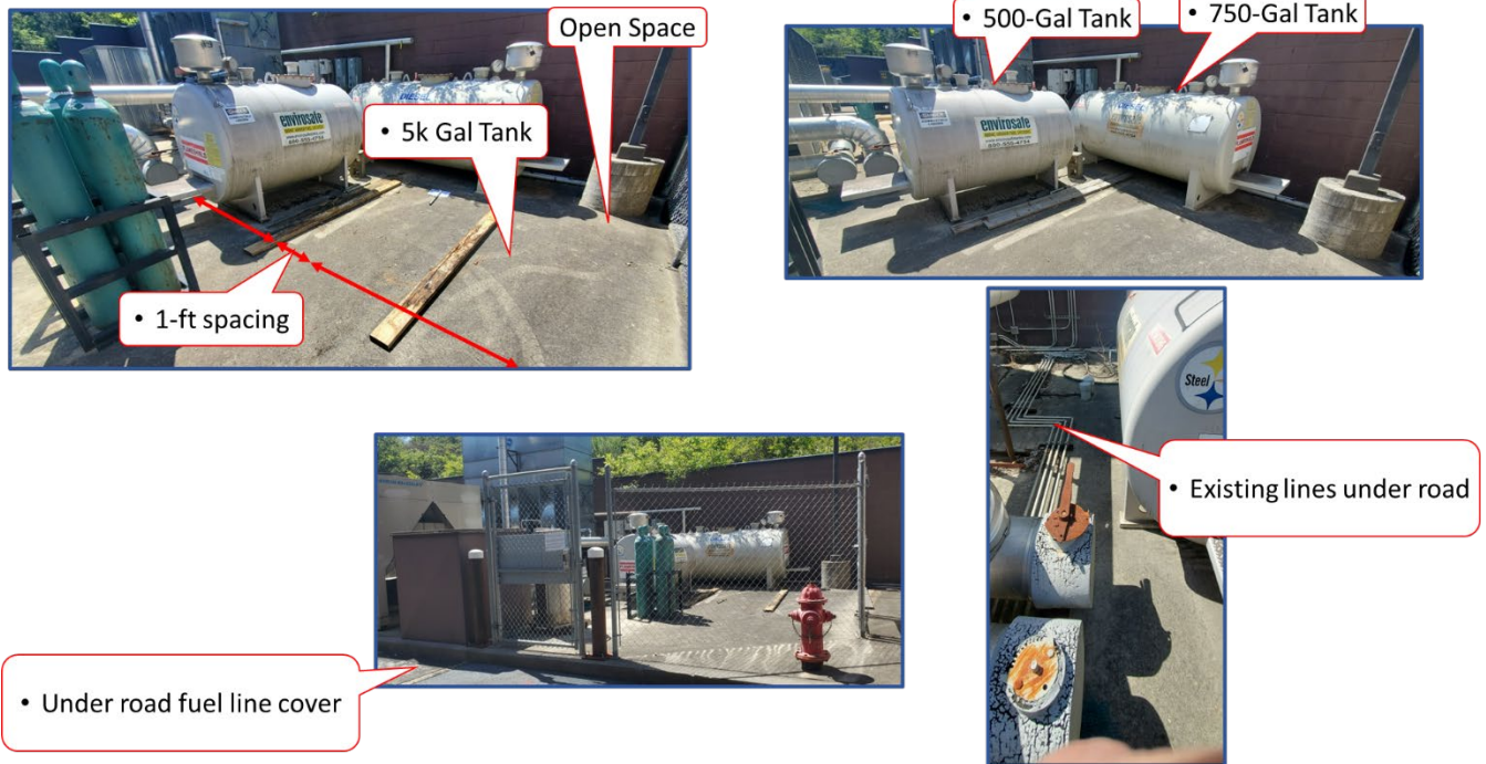
Figure 2. Fuel cage pictures where the 5000 (5k) gallon tank installation will occur.
