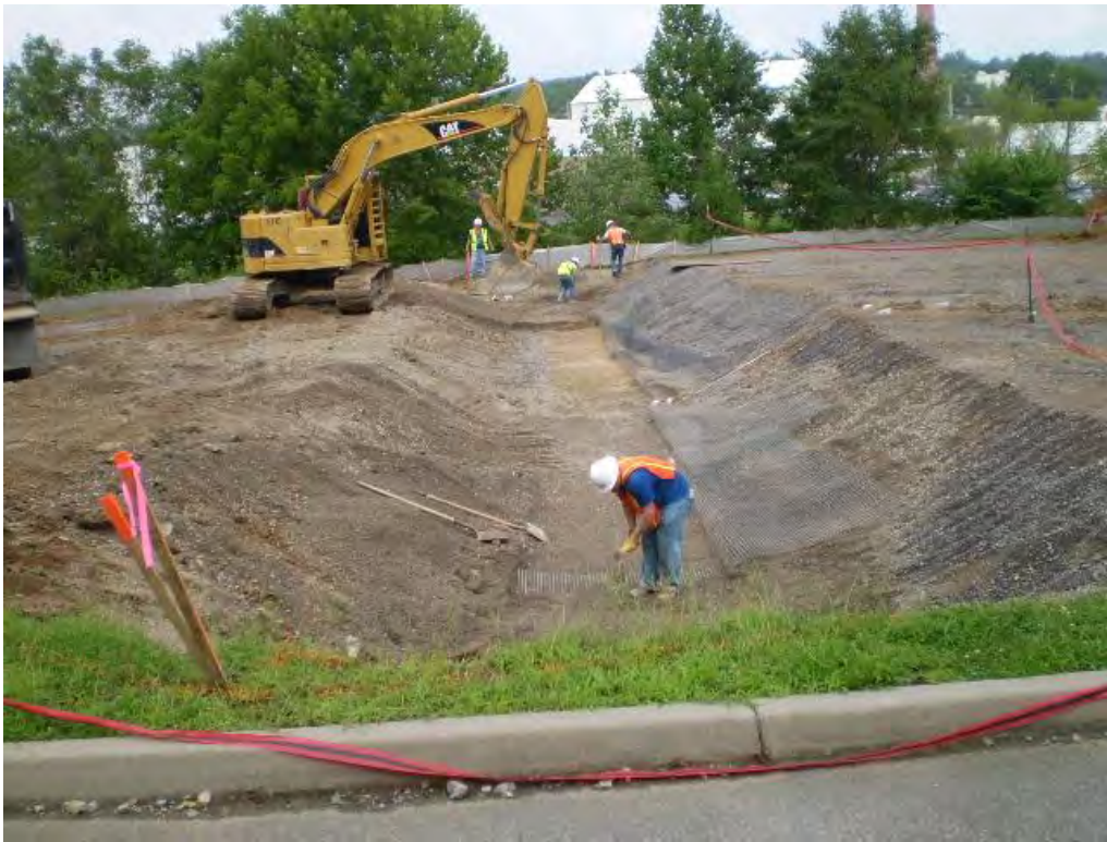
Photo 1 - View of undercut in main building area during excavation looking north 08-12-200. Note upper layer of existing geogrid is exposed and folded back on slope.
