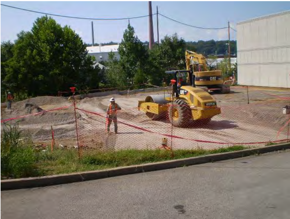
Photo 14 - View of large smooth-drum vibratory compactor used to compact mineral aggregate base backfill looking north 08-26-2009.
