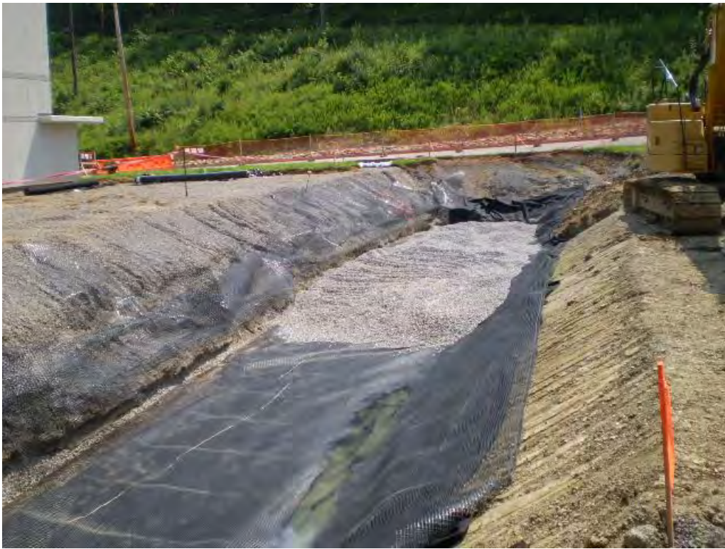
Photo 9 - View of no. 57 stone being placed in bottom of undercut in main building area looking south 08-25-2009.
