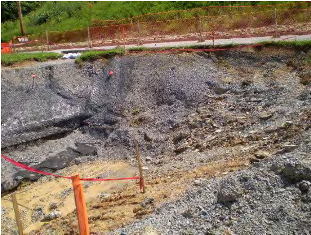
Photo 7 - View of limestone bedrock layers exposed in southern end of main building area undercut looking southeast 08-24-2009.
