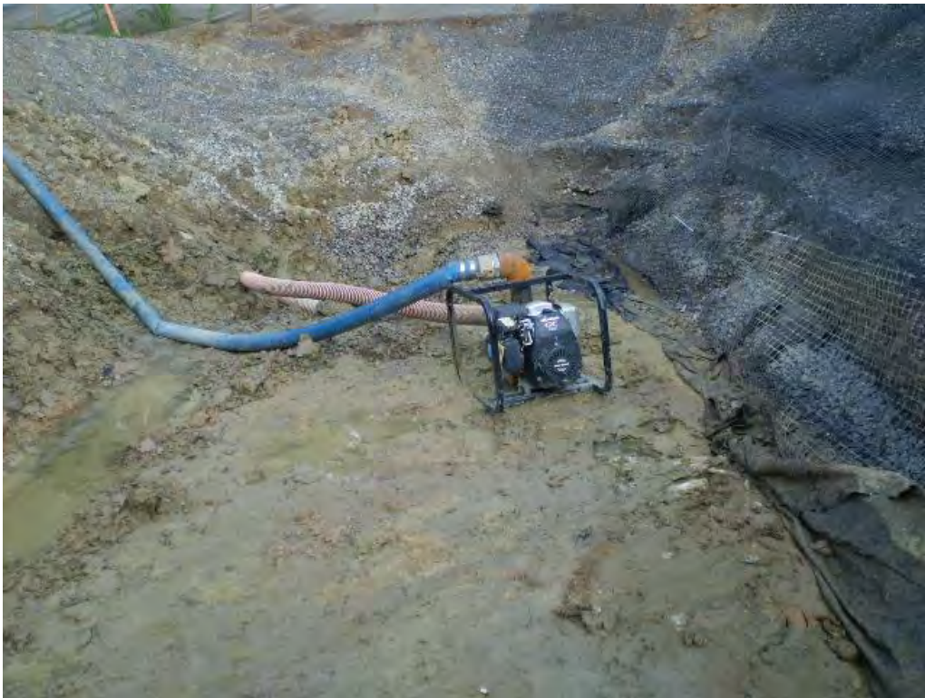
Photo 6 - View of sump pump operating in northern end of excavation in main building area to remove “perched” groundwater looking north 08-24-2009.
