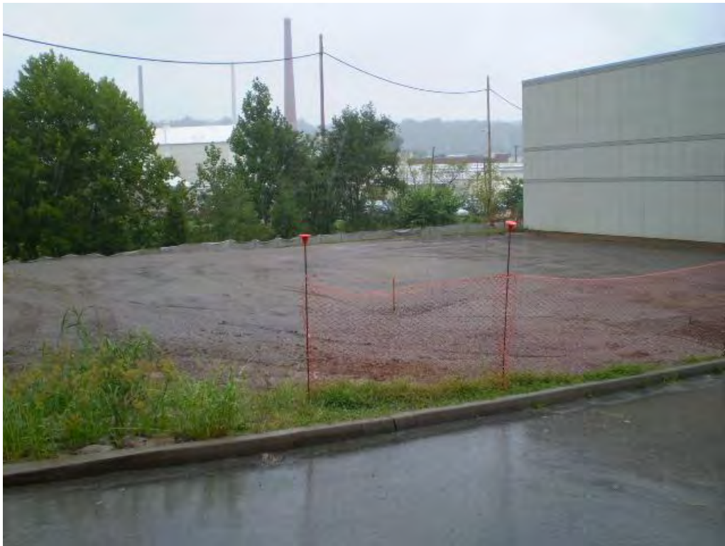
Photo 18 - View of site after new building pad is complete looking north 08-27-2009.
