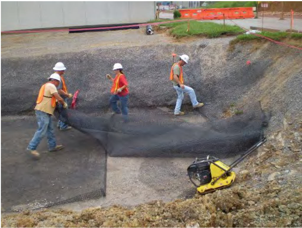
Photo 11 - View of workers placing second layer of geogrid in southern end of main building area undercut looking east 08-25-2009.
