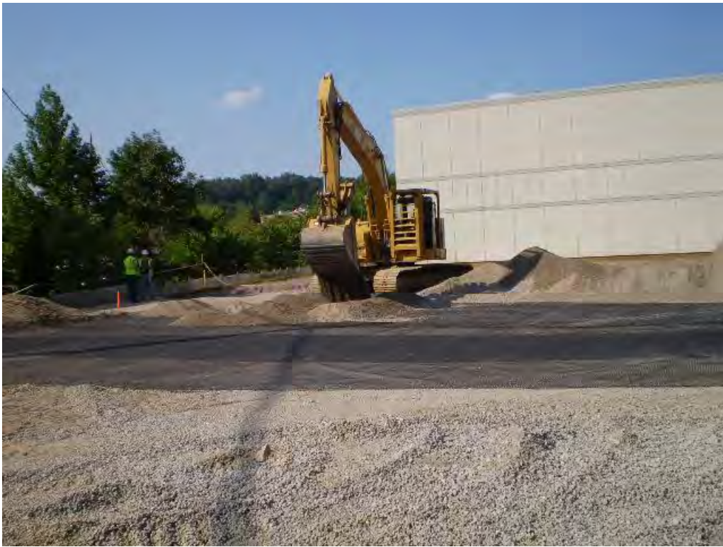
Photo 17 - View of trackhoe placing mineral aggregate base over geogrid in office/service building area looking northeast 08-26-2009.
