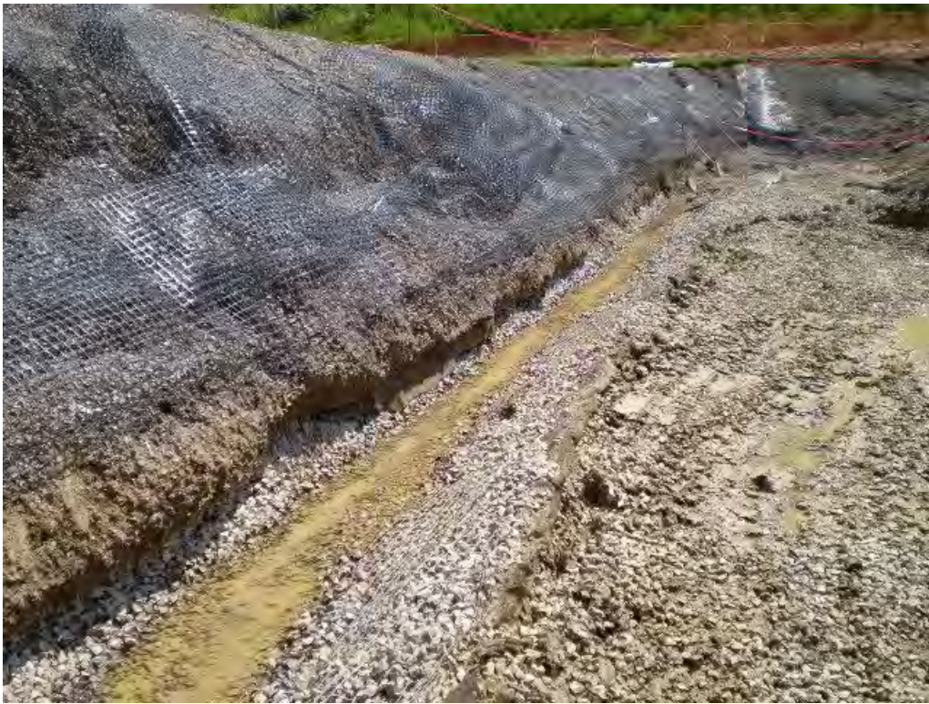
Photo 5 - View of undercut in main building area during excavation looking south 08-24-2009. Note existing basal layer of No. 57 Stone has been exposed and “perched” groundwater is draining from the stone.
