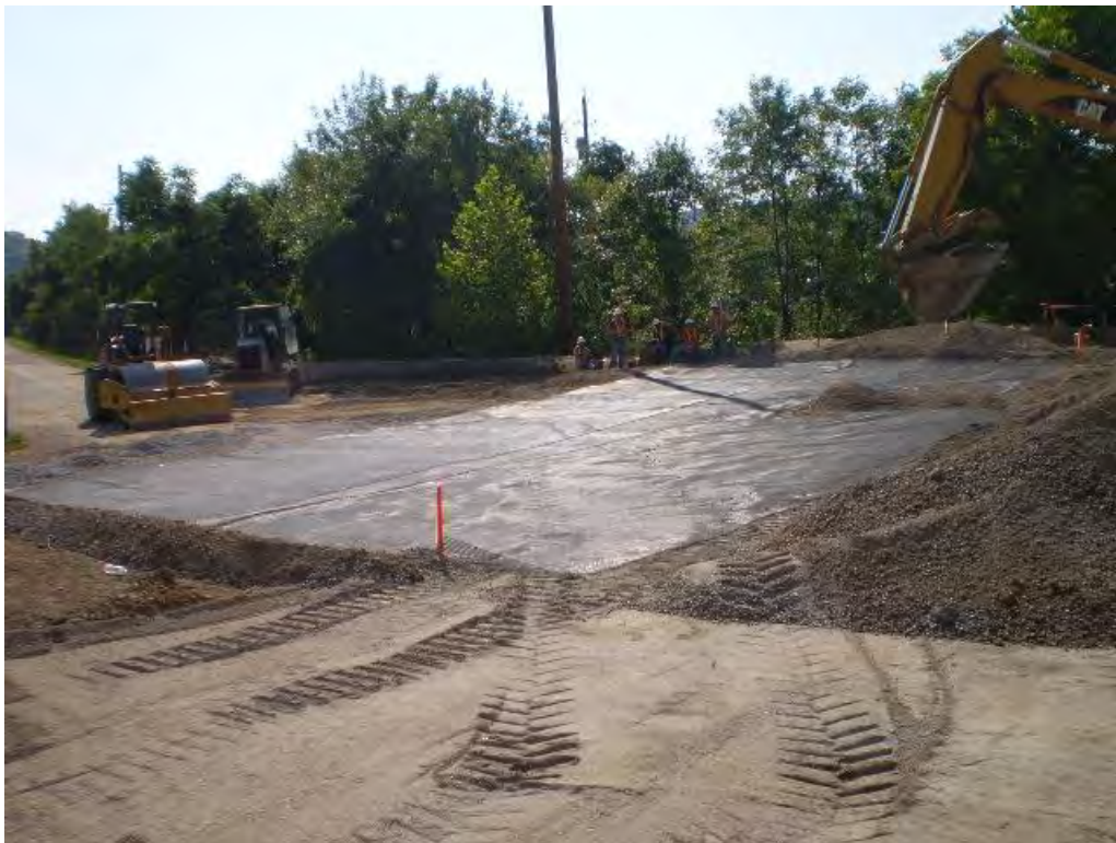
Photo 16 - View of office/service building area after placement of geogrid on prepared subgrade looking northwest 08-26-2009.
