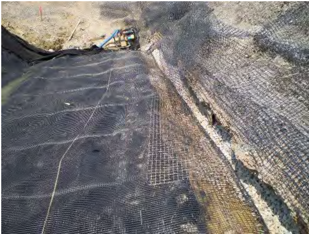
Photo 8 - View of geotextile and first layer of geogrid placed beneath main building area looking north 08-25-2009.
