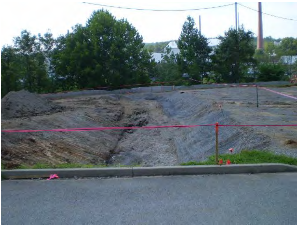
Photo 3 - View of undercut in main building area during excavation looking north 08-14-2009. Multiple layers of existing geogrid have been exposed and folded back on slope.
