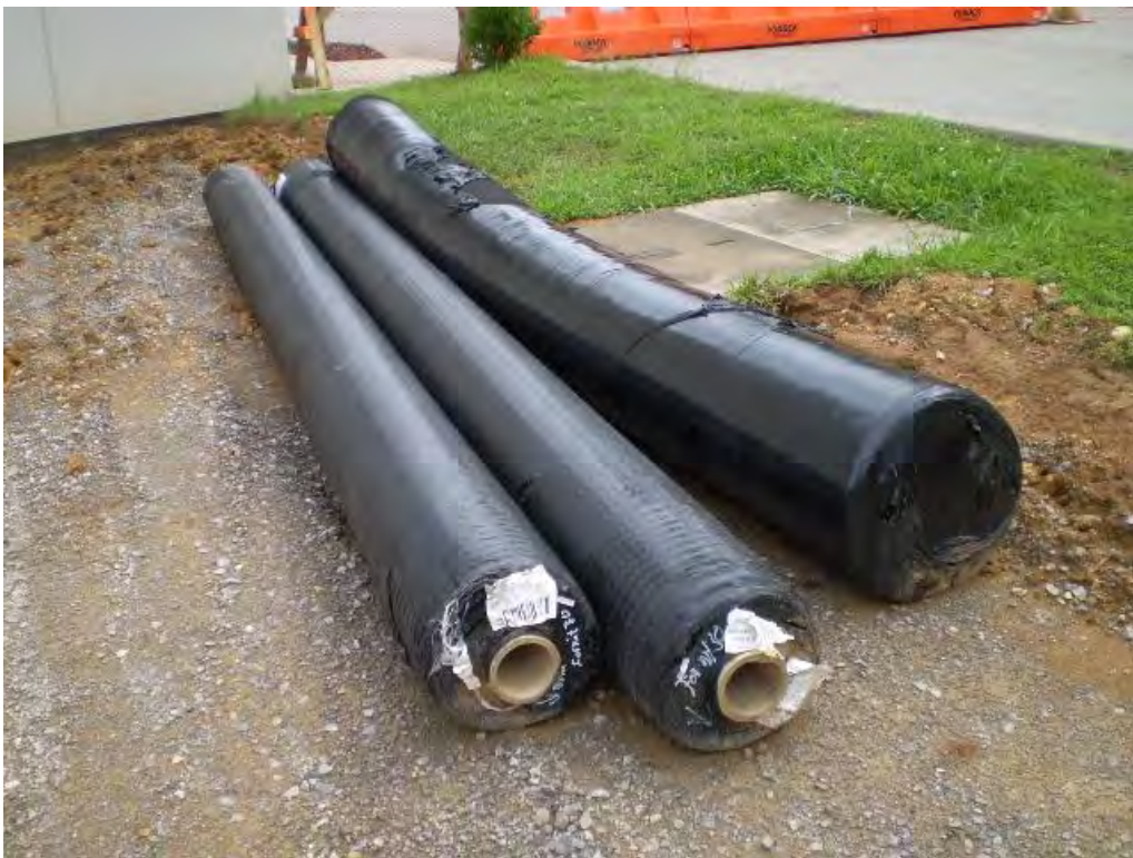
Photo 2 - View of rolls of geogrid and geotextile delivered to site 08-12-2009.
