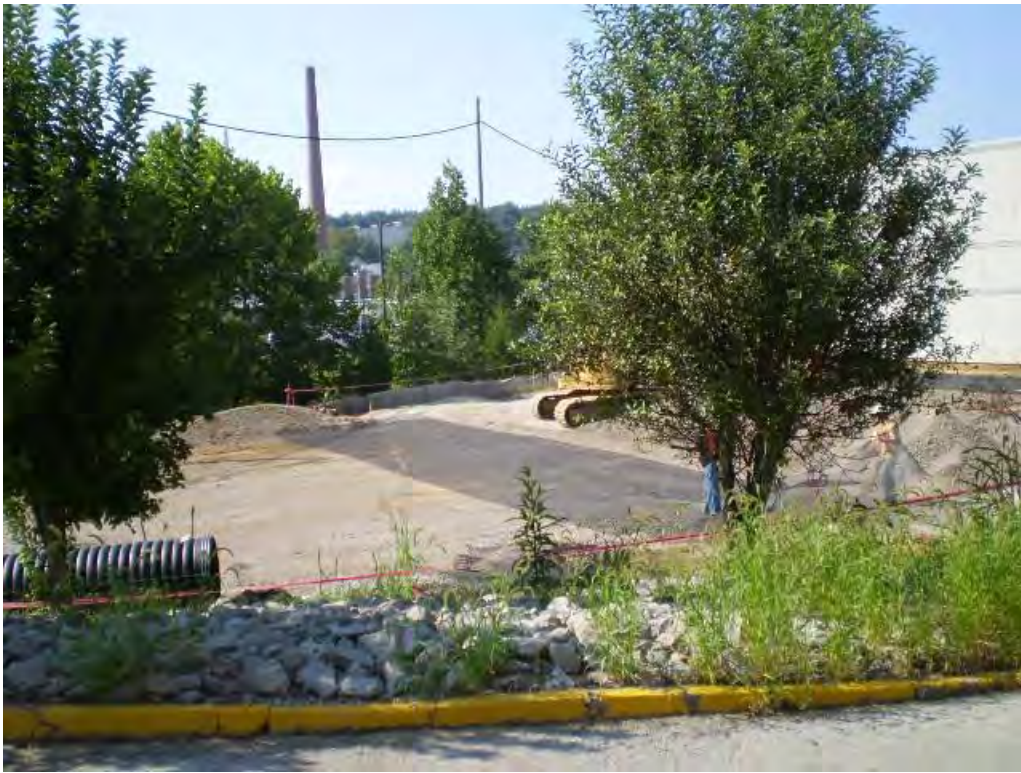
Photo 15 - View of main building area undercut after placement of third (last) layer of geogrid looking north 08-26-2009.
