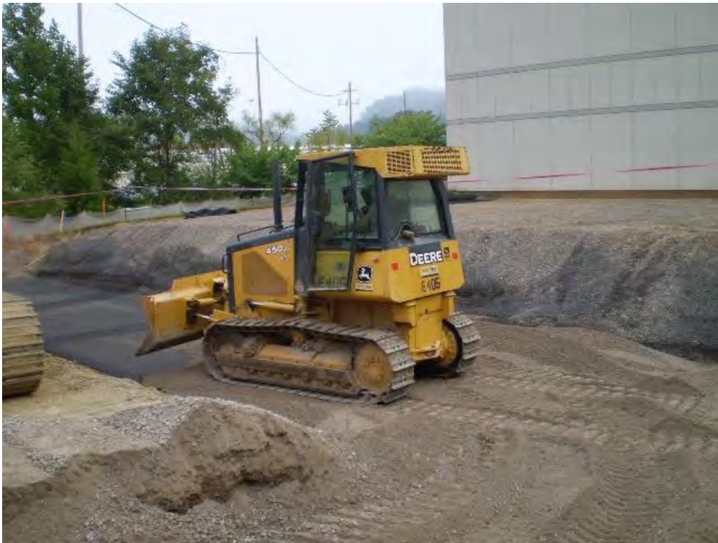
Photo 12 - View of small dozer spreading mineral aggregate base over second layer of geogrid below main building area looking northeast 08-25-2009.
