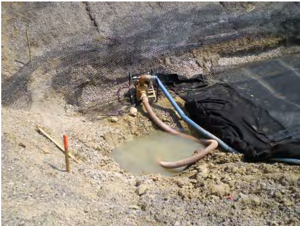
Photo 10 - View of sump pump operating in northern end of main building area undercut looking east 08-25-2009.
