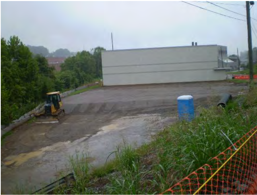
Photo 19 - View of site after new building pad is complete looking east 08-27-2009.
