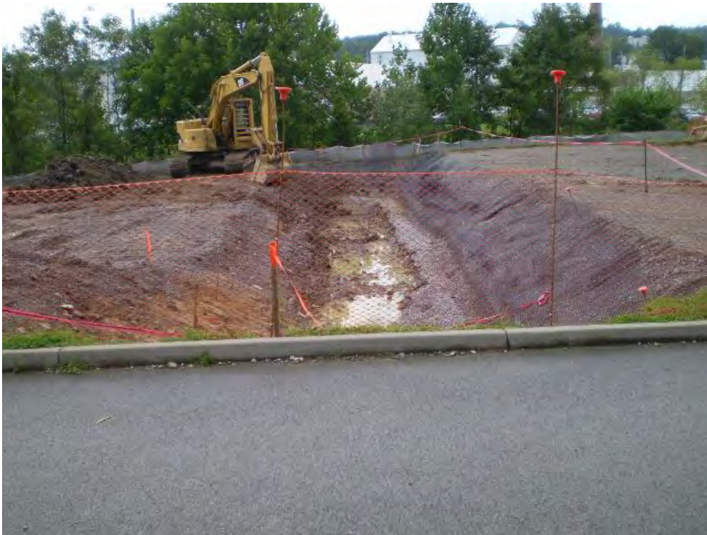
Photo 4 - View of undercut in main building area during excavation looking north 08-20-2009. Site received rain this afternoon prior to making photo and rain water has accumulated in the excavation.
