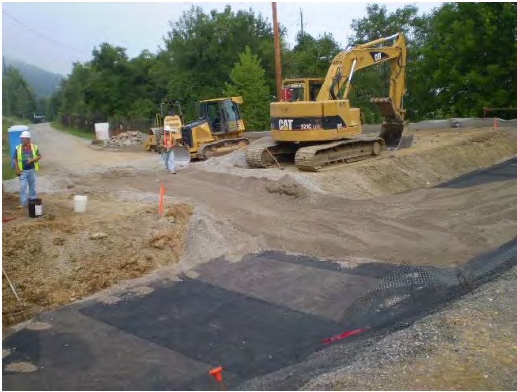
Photo 13 - View of undercut in main building area during placement of mineral aggregate base over second layer of geogrid looking west 08-25-2009. Note ramp excavated previously to provide access for backfilling.
