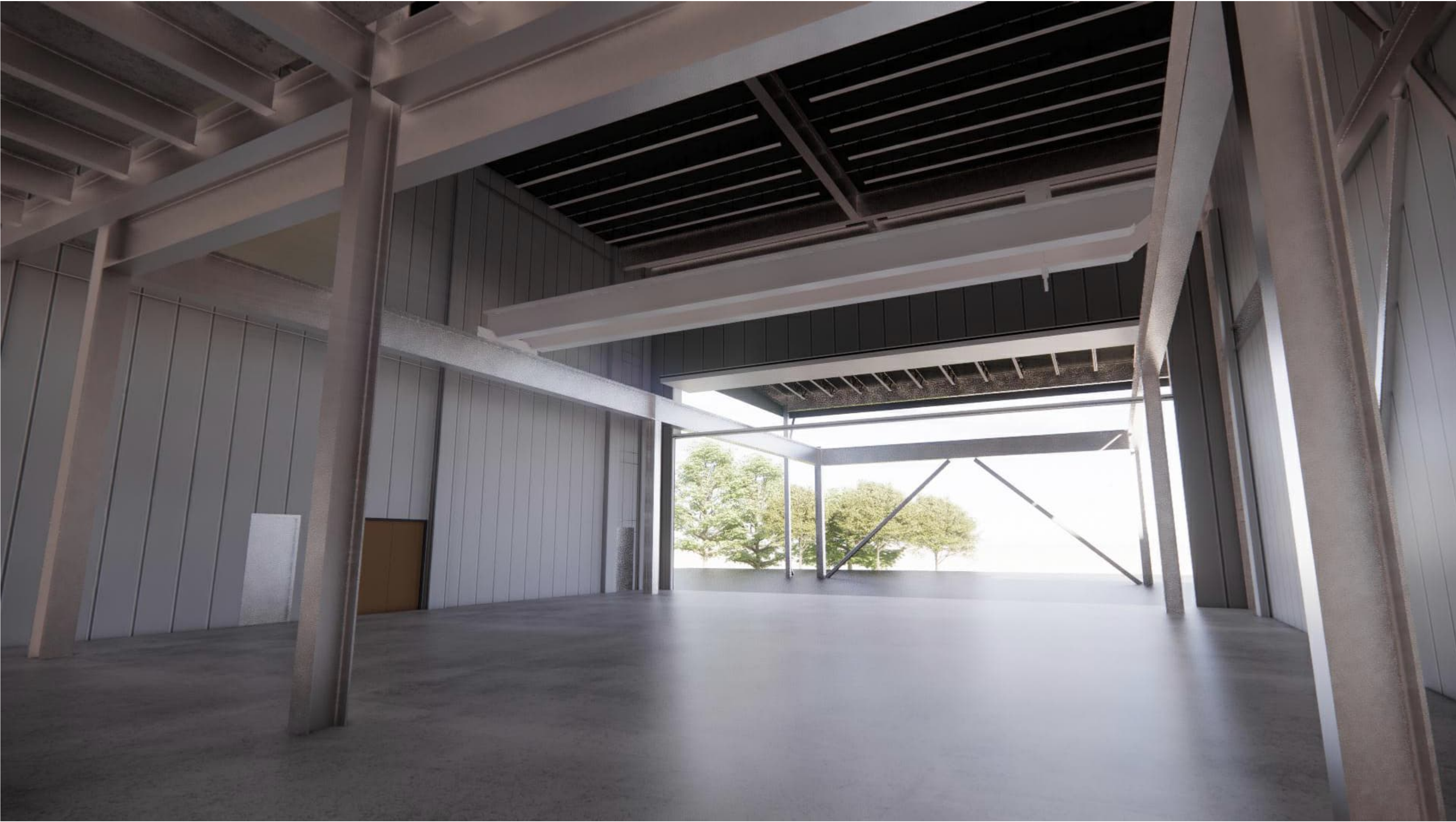
VIEW OF TRUCK BAY
